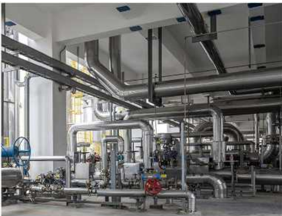
Dual -cam in pipeline inspection
